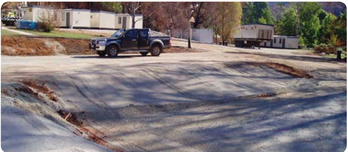
Marysville Temporary Village under construction, March 2009
