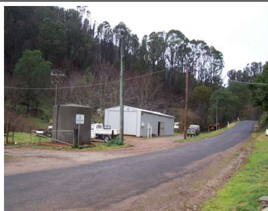
Additional works are planned at Gaffneys Creek where a 22,000 litre water tank has recently been provided adjacent to the Community Meeting 'Shed' to support fire fighting purposes.
