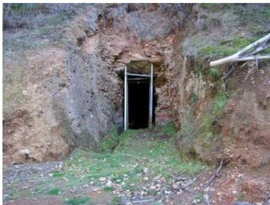
Pre upgrade condition of Mine Adit /Fire Refuge
